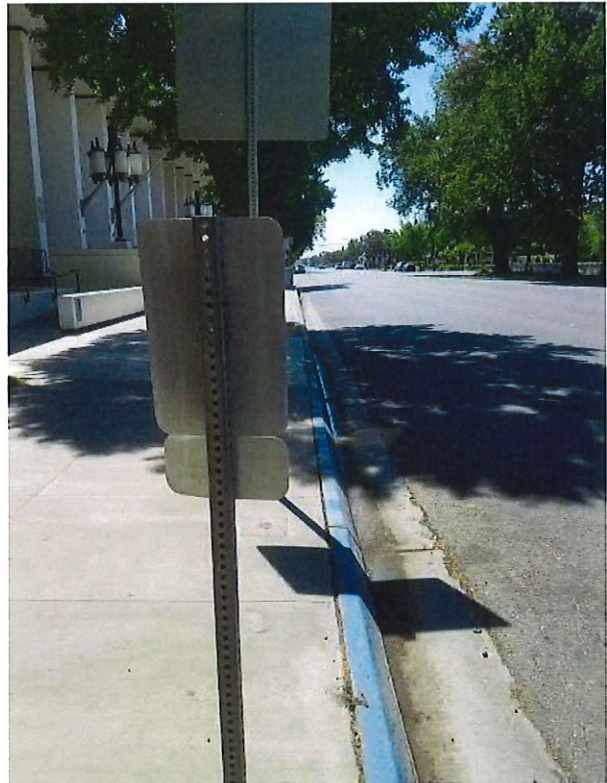
Graffiti, weeds and gutter all cleaned at the Library. (After)
